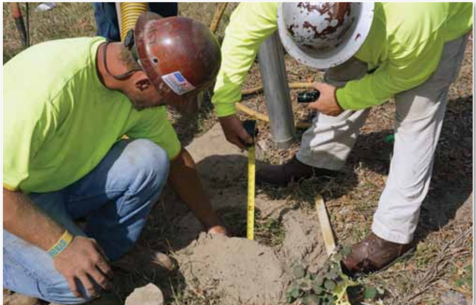
Measuring the depth of a verified utility.
