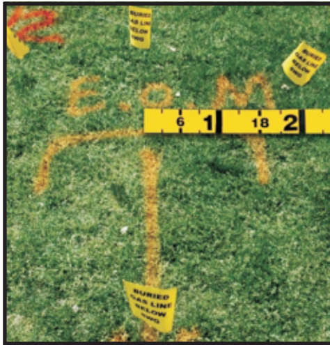
Document the markings before you dig
