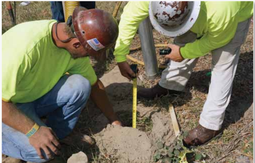
Measuring the depth of a verified utility.
